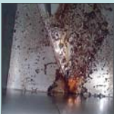
Sludge in tank
